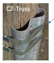
C2-Truss: used primarily for reinforcing distribution poles.
