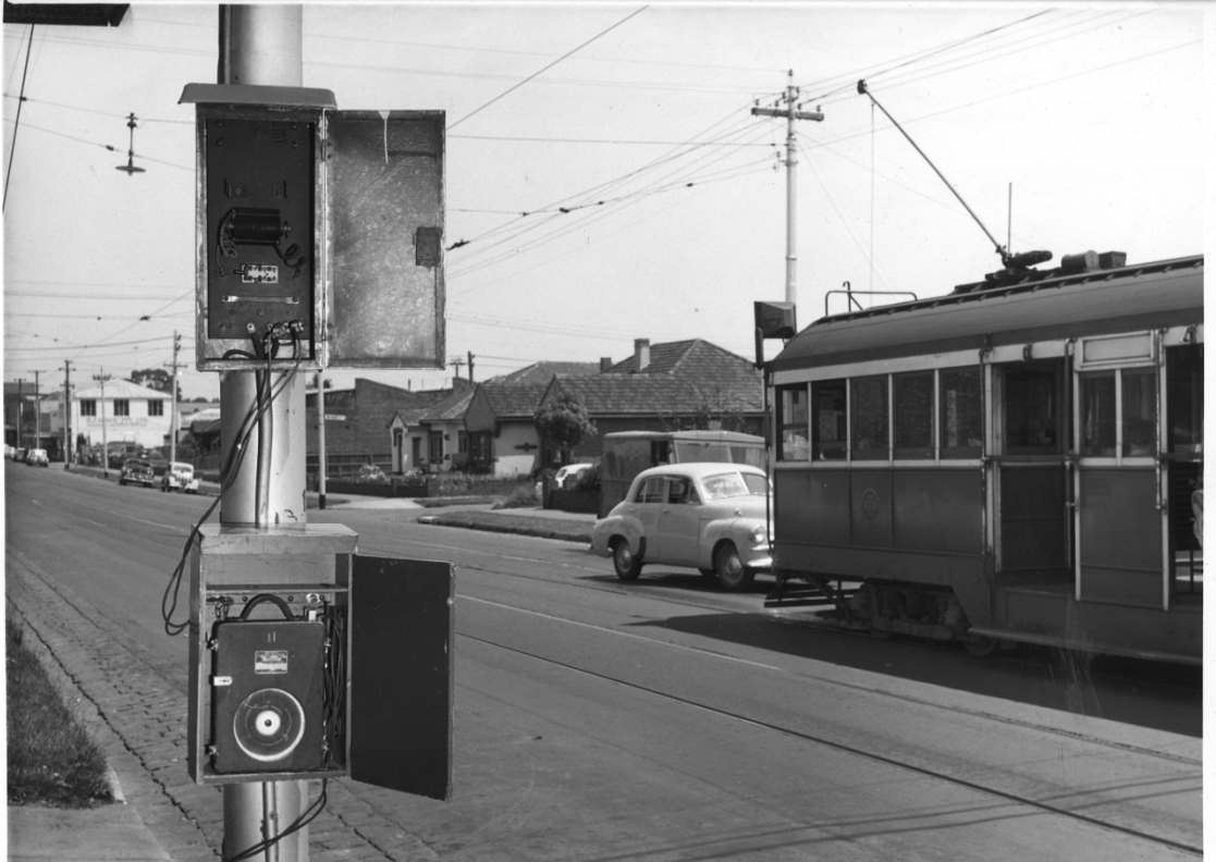
12.3 Drainage Bond Opposite Glenhuntly Tram Depot
