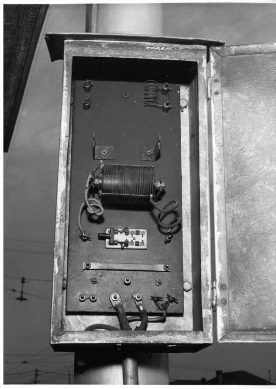
12.7 MMTB Unboosted Drainage Bond
