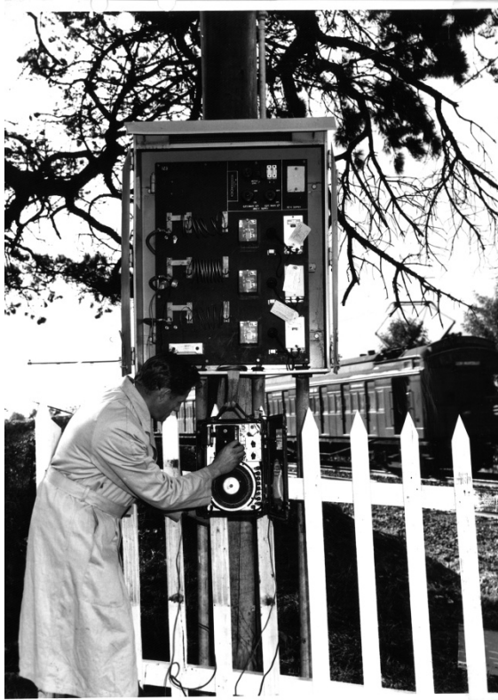
12.14 VR Drainage Bond – Bristol Recorder
