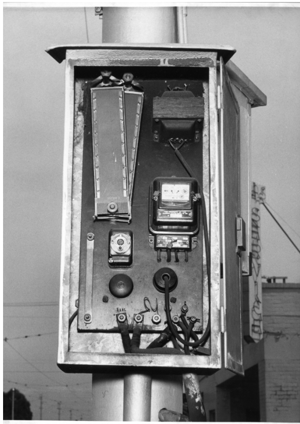
12.6 MMTB Boosted Drainage Bond
