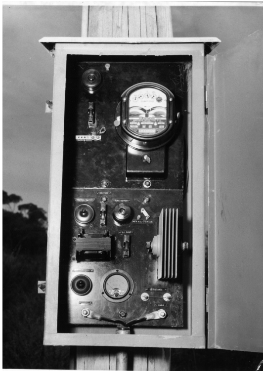
12.10 PMG CPU – Geelong Road at Werribee Bridge
