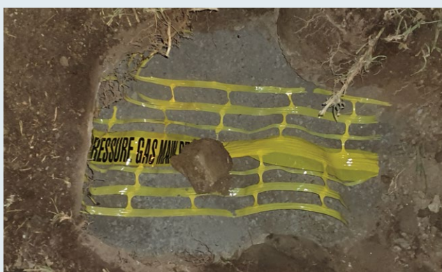
Figure 23: Yellow marker tape to provide warning of underground gas services
