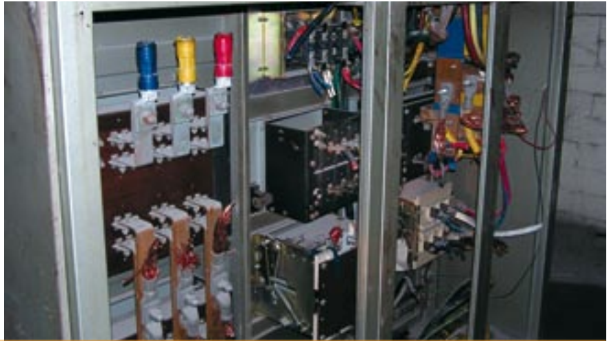
The main switchboard at a disused Yarraville factory. The back panels had been removed for thieves to steal copper. A 21-year-old "urban adventurer" suffered a severe electric shock and massive burns when he came into contact with the switchboard (See this page).
